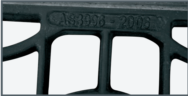
Cast iron or galvanized wave grate to AS 3996-2006.
